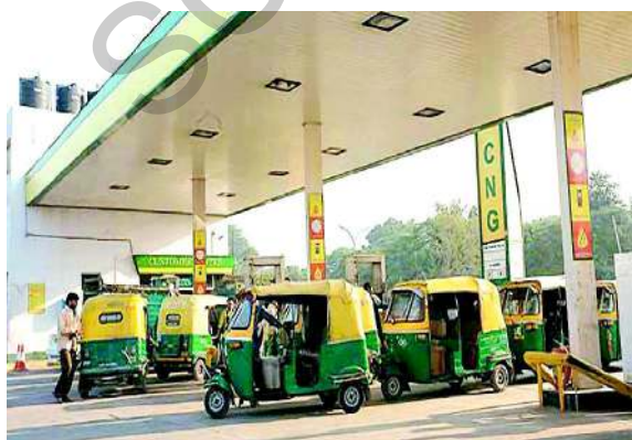
Fig - 3: CNG filling station
